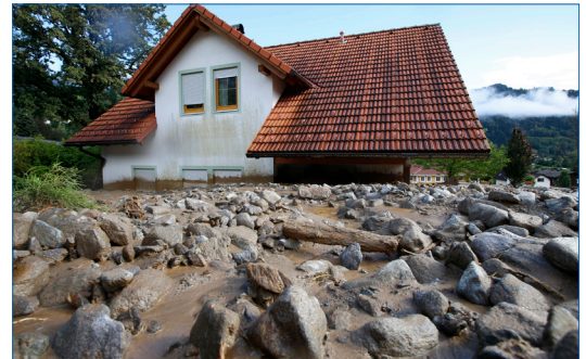
Debris flow in Aflritz, Carinthia, August 2016 © Photo: BMNT/ WLV
