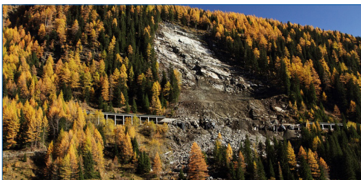
Rockslide destroyed protection tunnel, East Tyrol, 2013 © Photo: Martin Mergili
