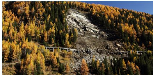
Rockslide destroyed protection tunnel, East Tyrol, 2013
